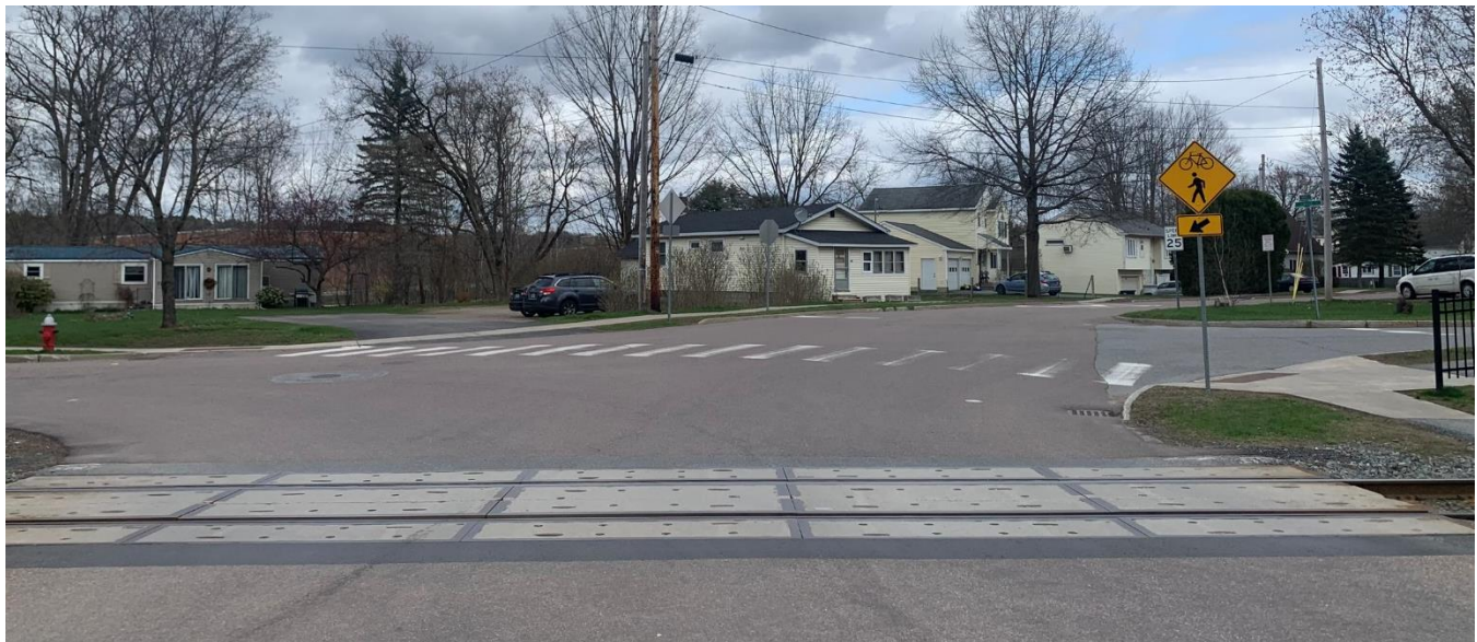
Figure 3: North Street/Grove Street current conditions (photographed 4/14/2024)
