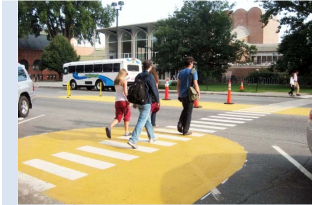
Temporary Bulb-out in Hanover, NH
