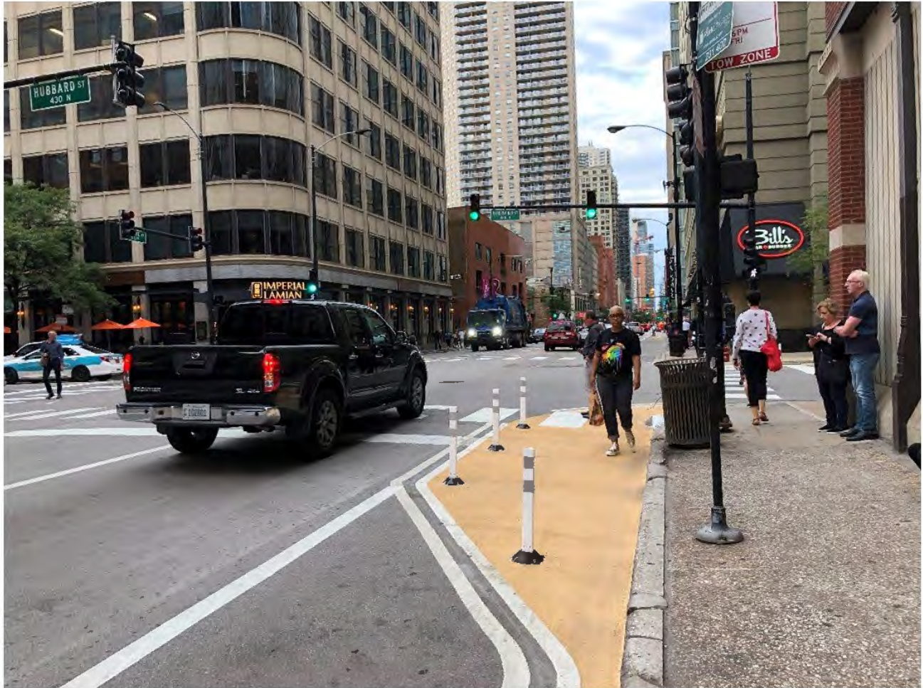
Figure 8: Temporary curb extension in Chicago, IL
