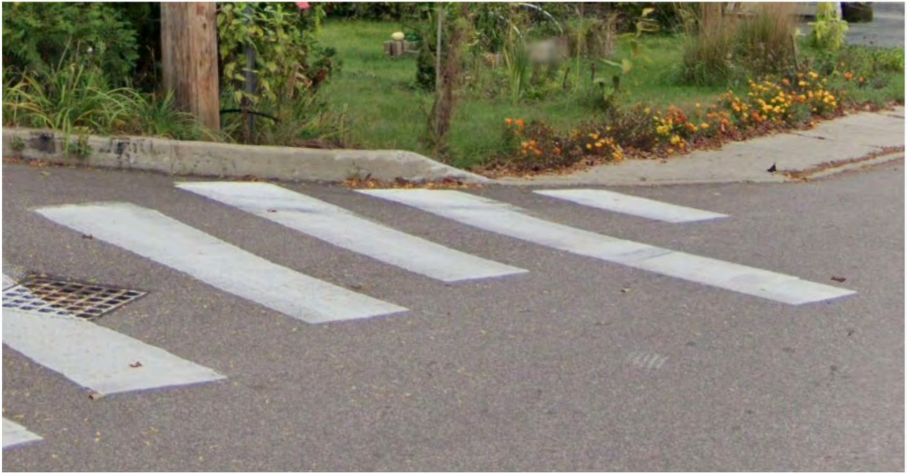
Figure 2: Street view of elongated vehicle stop bar conflicting with crosswalk striping. Source: Google street view
