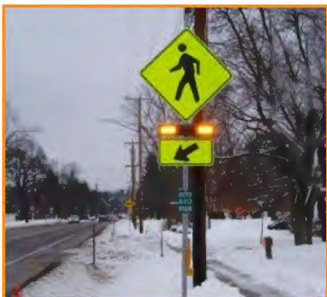
Rectangular Rapid Flashing Beacons alert drivers to pedestrians in the crosswalk.
