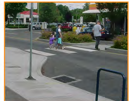
Curb Extensions help slow traffic at crosswalks.
